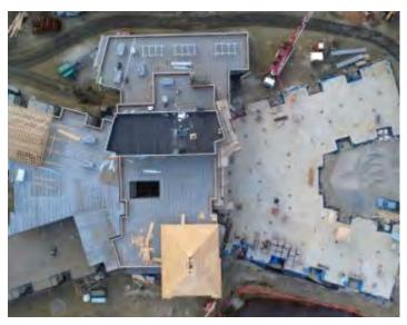
A Wing – all steel has been erected and west wing stairs – structural steel in place. B Wing – slab on grade poured and ready for structural steel, which is scheduled to be delivered next week.
